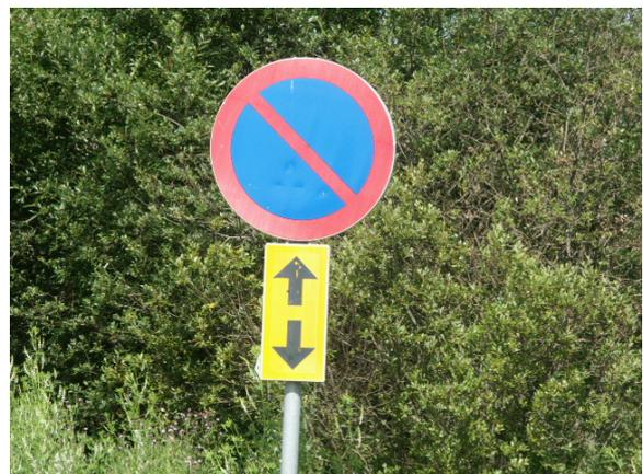
Figure 1.7: Faded Traffic Signs [20]
