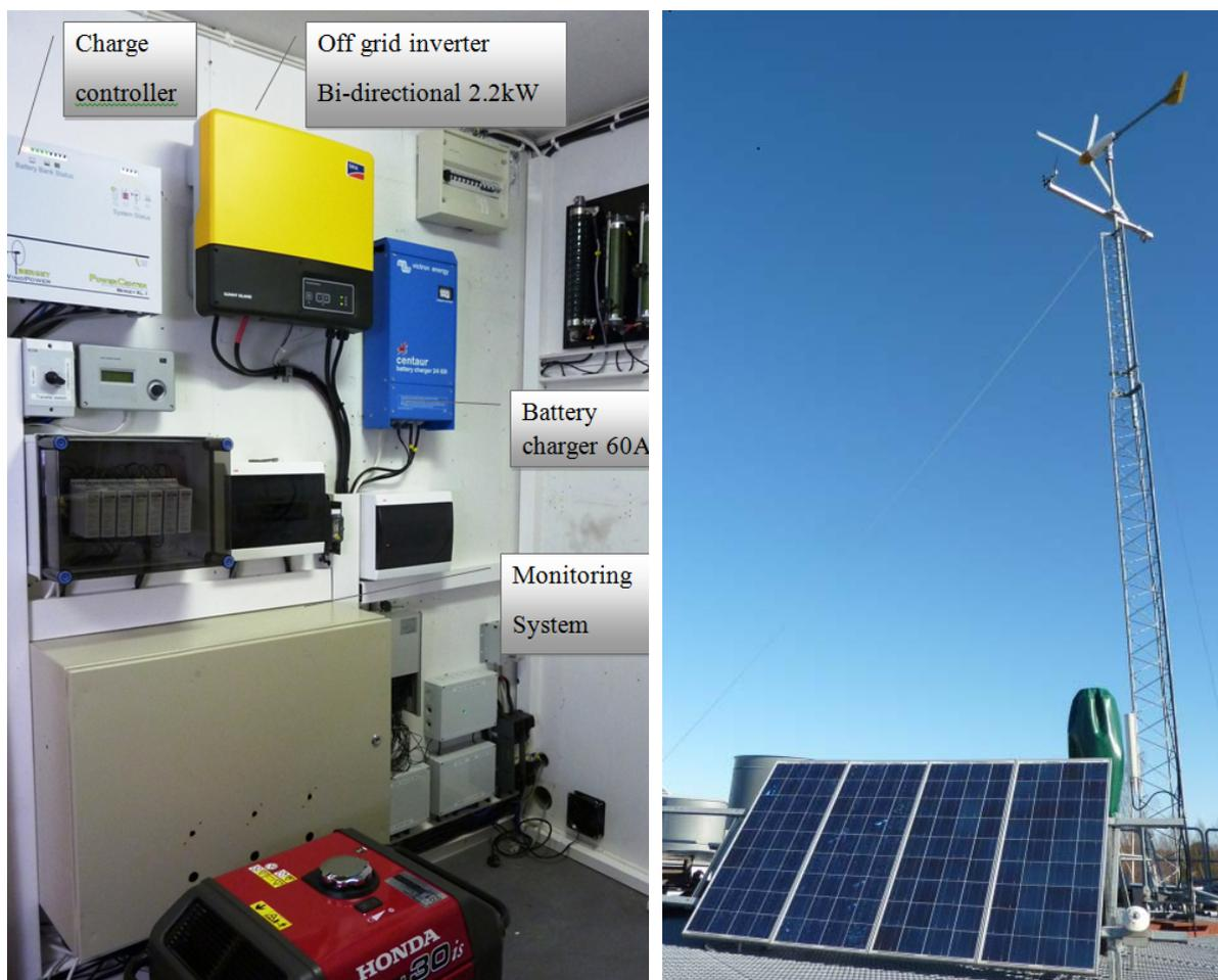
Figure 2: Indoor (left) and outdoor (right) equipment of the testing and demonstration facility.
